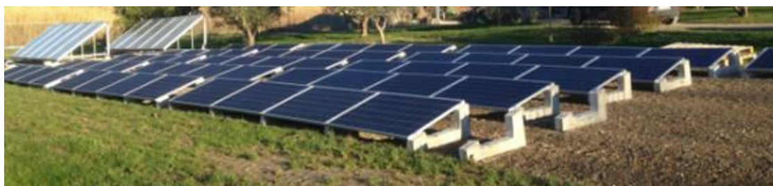
Figure 19: Design of the photovoltaic plant on the ballast fixing structure
