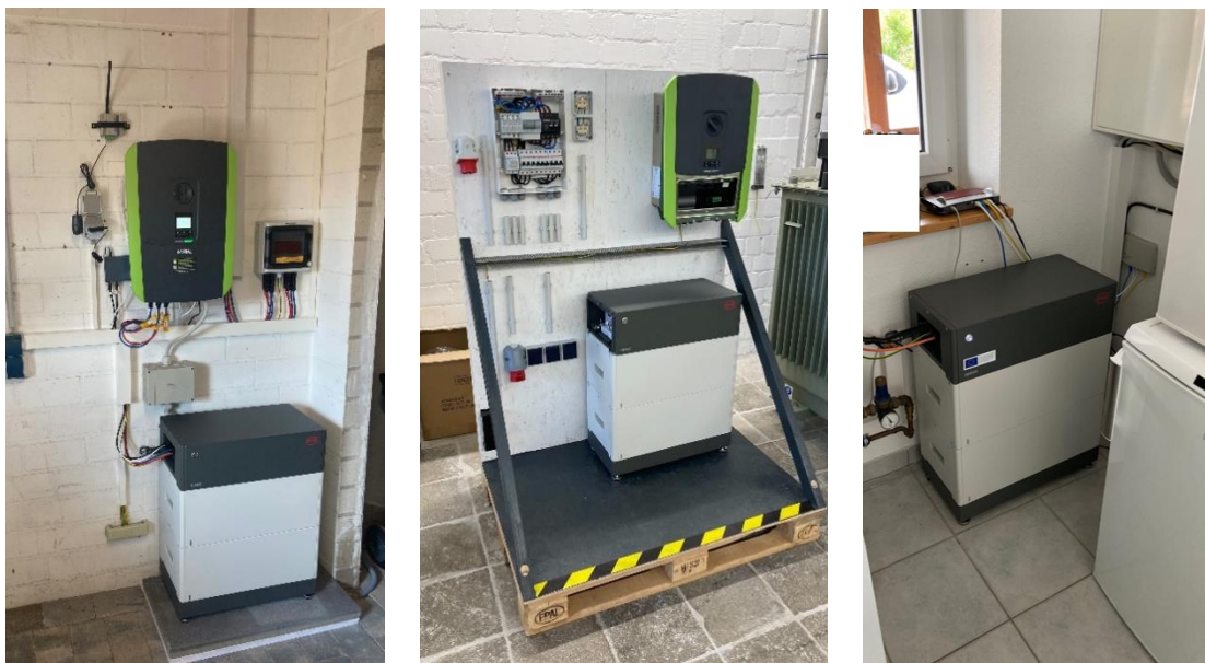
Figure 12: Residential HBES system and HBES system prototype
