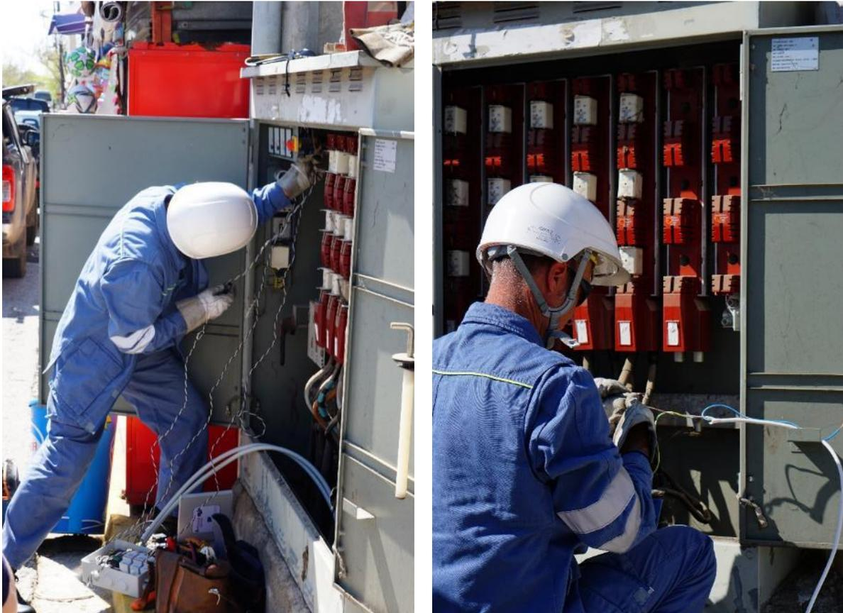
**Figure 31: Connection of current signals (left) and preparation for connection of voltage signals (right) in MT02 substation.**
