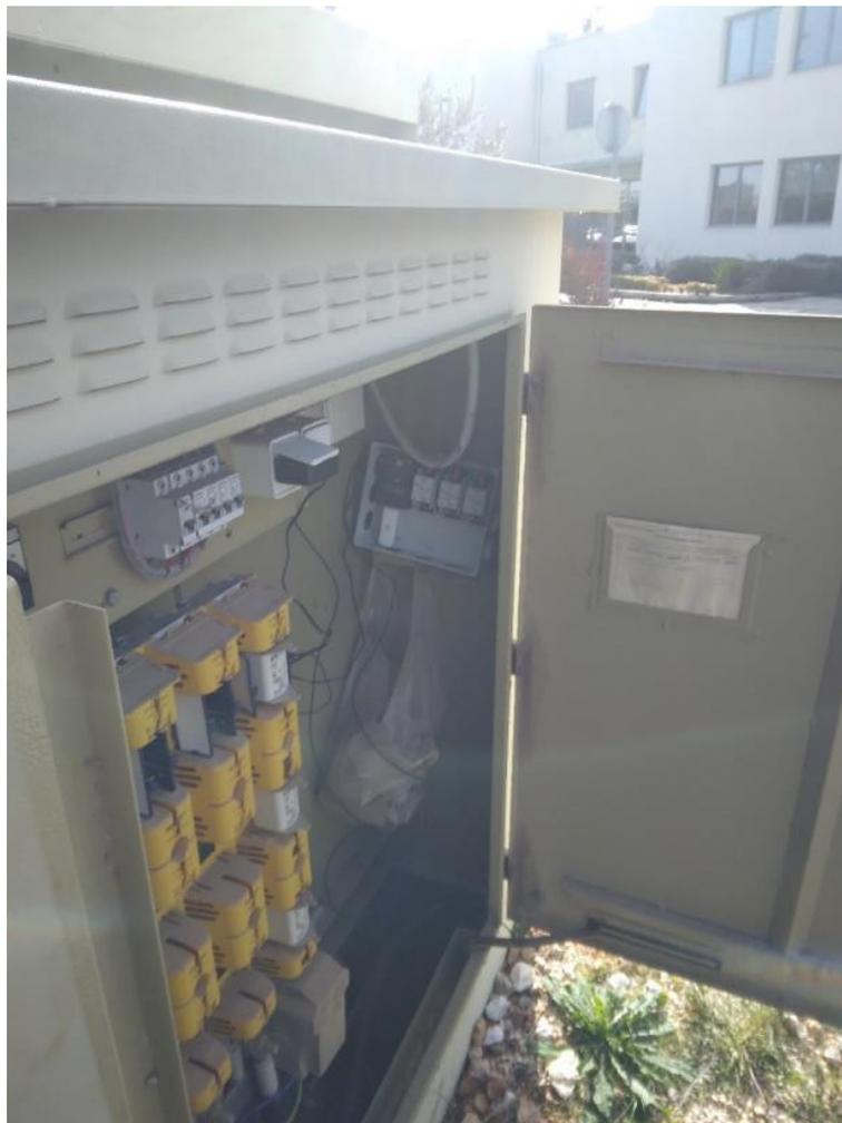
Figure 30: Trial placement inside the MV/LV pillar.
