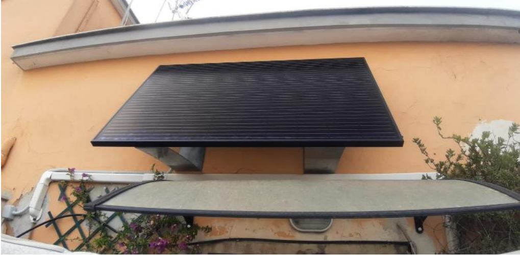
Figure 24: 250W PV plant
